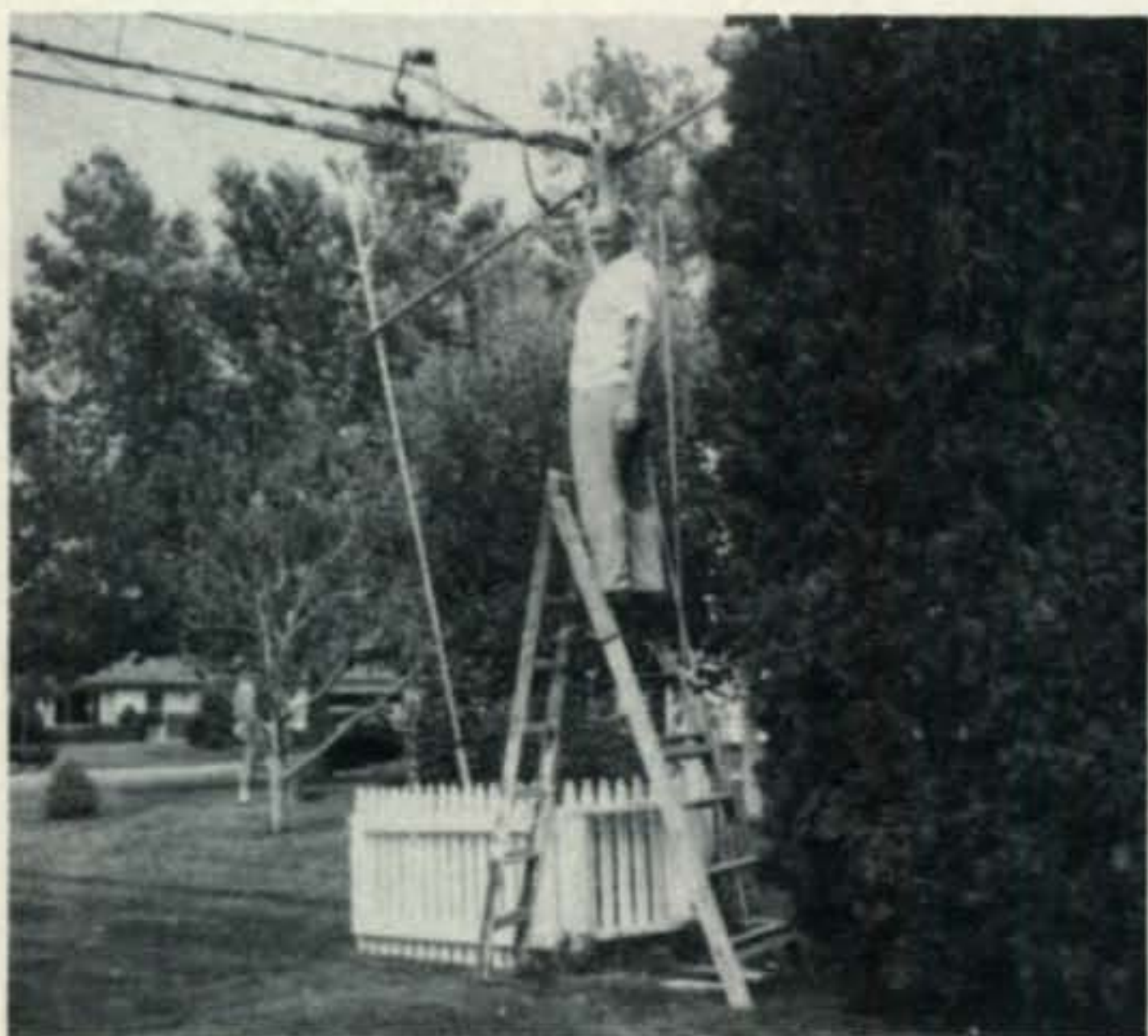
Fig. 1—Tower in the down position. The final height above ground depends on the antenna.
