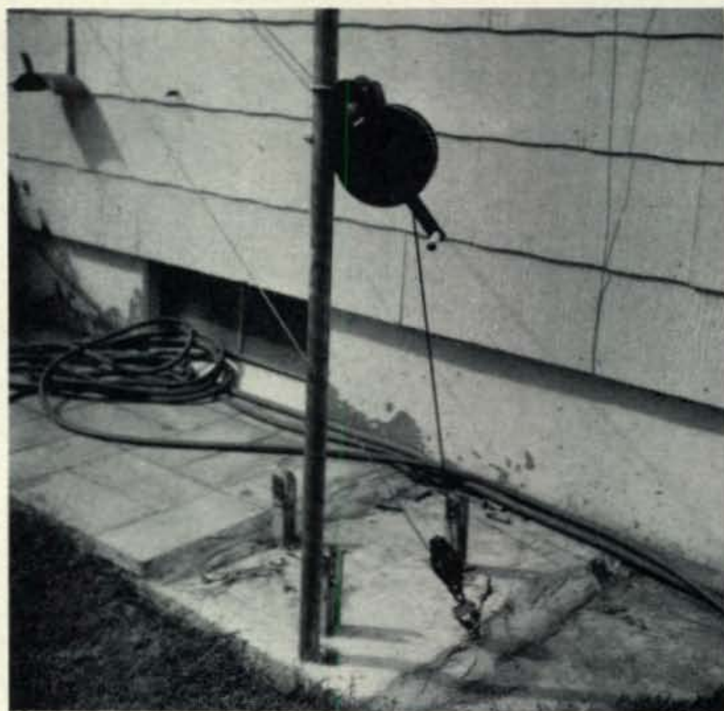
Fig. 3—A 1600 pound double locking boat hoist from Sears Roebuck does the job, along with 3/16" galvanized cable, a 750 lb. pulley, and a 1/2" eyebolt in 4 feet of concrete.
