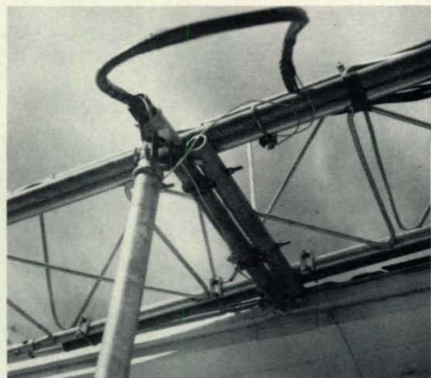
Fig. 4—The tilt-over mechanism is based on 3 muffler clamps which rotate around the horizontal part of the 1 1/4" pipe. These are attached to another piece of 1 1/4" pipe. This latter piece is attached to 1" reinforcing pipes (see fig. 6) attached to the tower.
